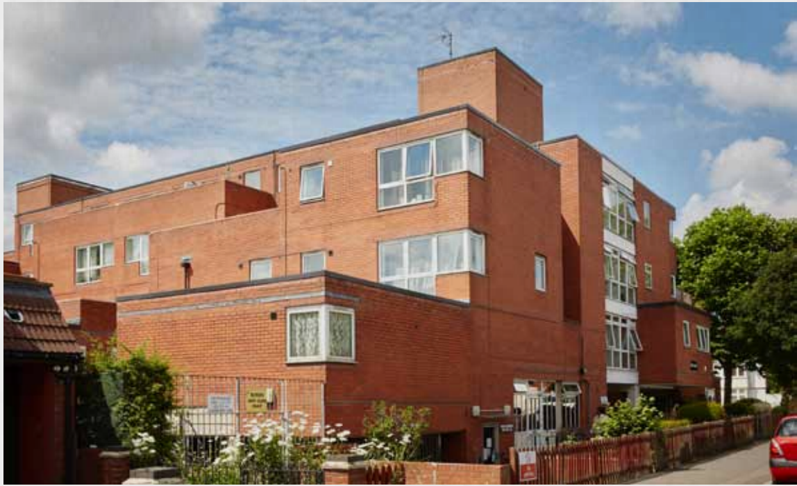
Libro Court had extensive improvement and repair works carried out.
