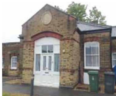
External redecorations were also carried out and all works were undertaken
