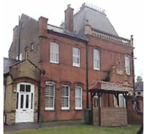
by contractor Woodbar Ltd as part of WFHA's planned maintenance programme.
